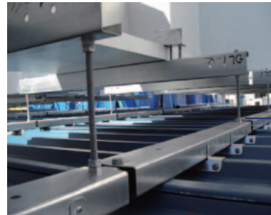
◀Pier Cover Plate Mounting
