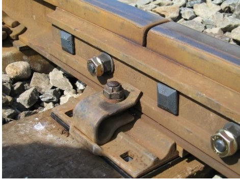
Fishplates (Japan Railway) Thick-Type M20 C8
