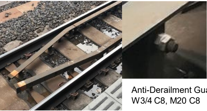
London Underground Adjustable Stretcher Bar M20 C8
