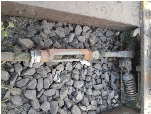
Turnbuckle for rail track HLN M30 SS400 & M30 Left handed * to ensure strengthen the track so that the rails are held in position
